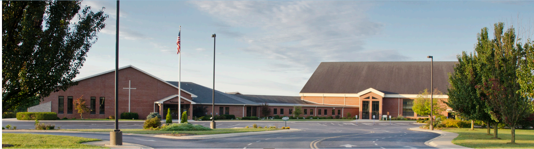
SHERWOOD OAKS' BUILDING, 2012
